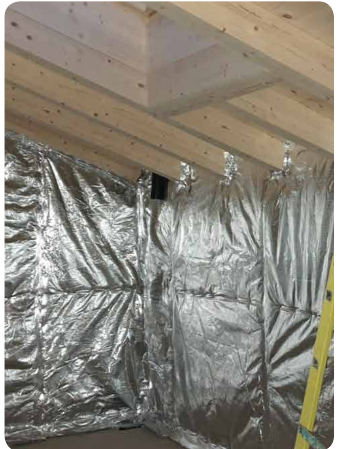
● Posa isolante Over-foil Multistrato 19
